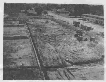
This is as of last Monday, and despite the slippery footing from Sunday's rains, the construction crew are hard at work putting in the big drain lines. Kind'a amazing to see that crane with a scoop on it picking up the huge tiles, and placing them as gently as a feather. After the ditches are filled, and the whole base filled with sand, the superstructure will start to go up. Messrs. BECKMAN, KEROUAC and TRAVIS are all "champing at the bit", ready to start using the place.
